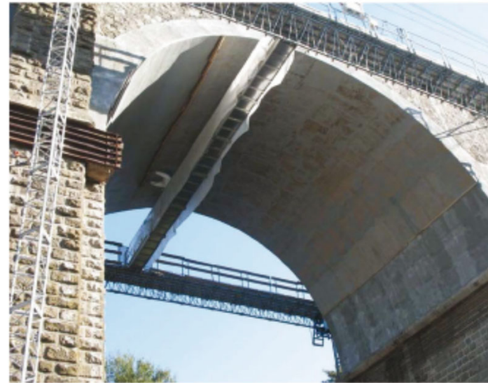
Fig. 4.1.2a—(a) Bridge structure with view of scaffolding; and (b) installation of FRCM.
